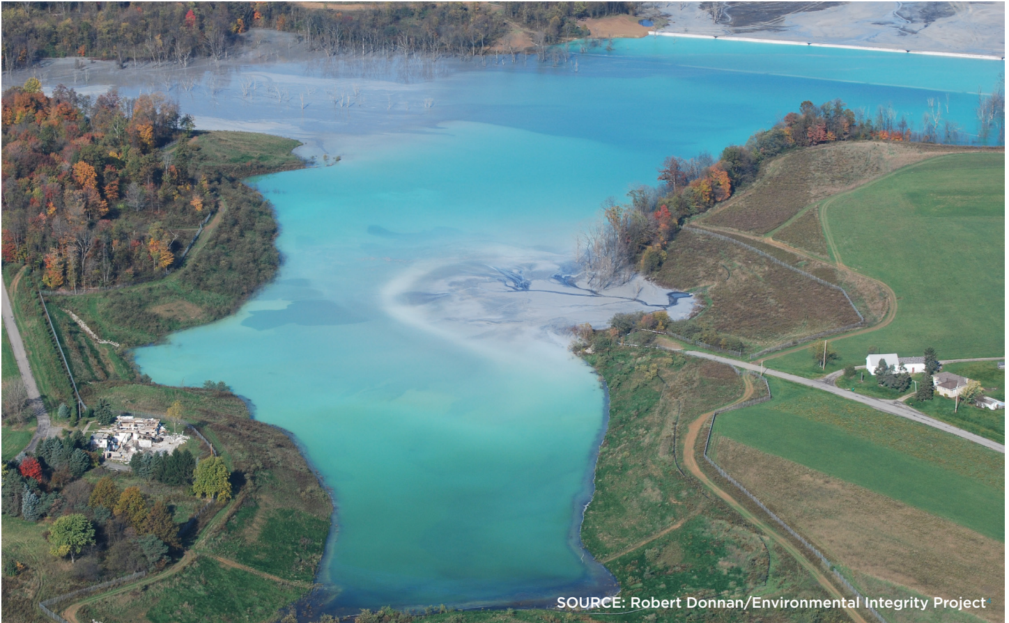
FIGURE 1: FirstEnergy's 967-acre Little Blue Run coal ash pond, one of the largest in the country. Under the terms of a successful lawsuit, it will have to be closed in 2016.
